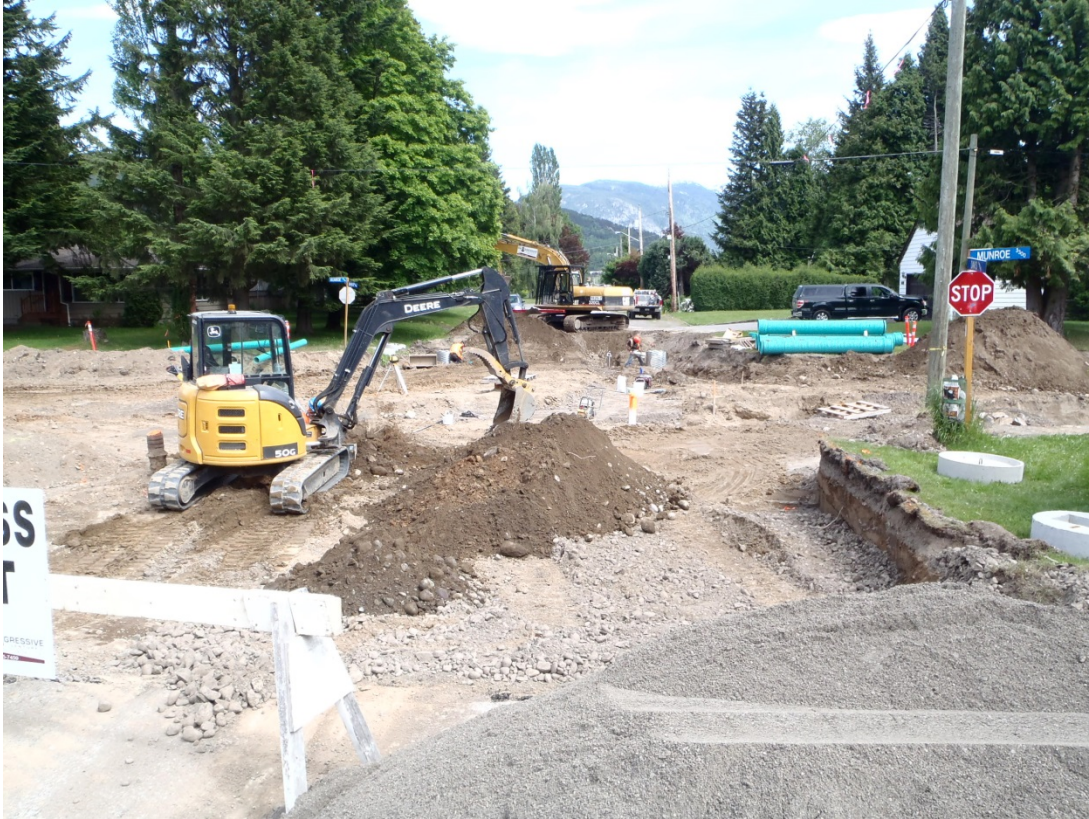
Figure 33: Munroe Street Road Construction Project
