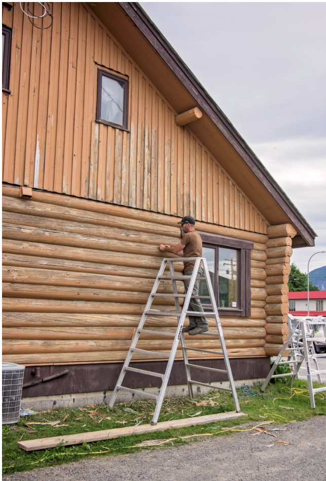
Figure 31: Work on the Visitor Information Centre
