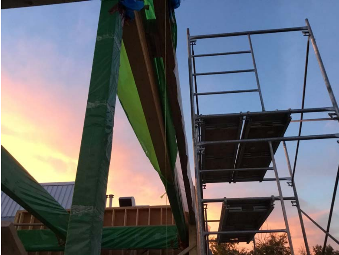
Figure 27: Scaffolding at the Terrace and District Aquatic Centre
