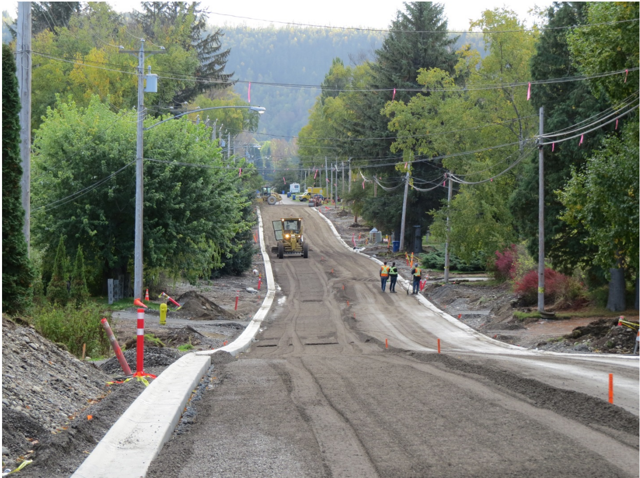
Figure 32: Kalum Street Road Construction Project
