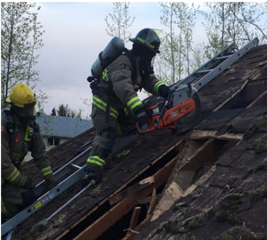
Figure 18: Fire Fighting in Action
