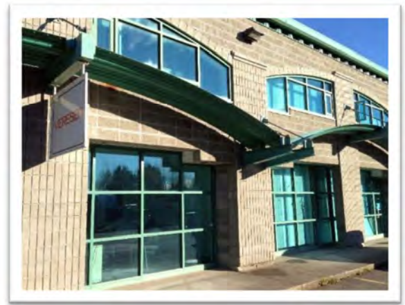
Example of High Transparency Light Industrial Building Facade
