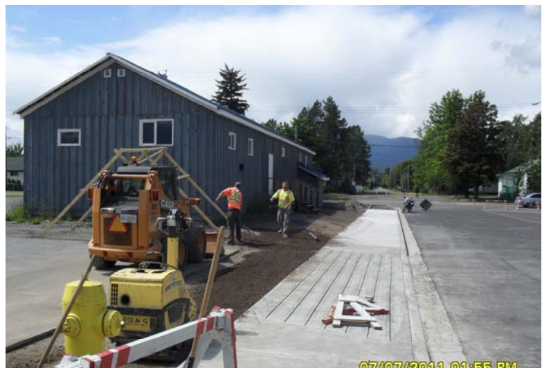
Rebuild of Davis Avenue
