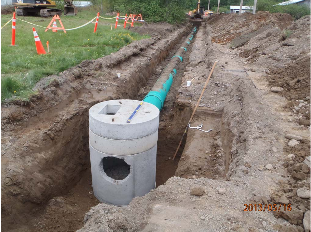
Reconstruction of 5000 Park Avenue
