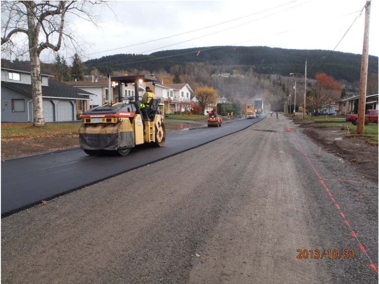
Road Reconstruction on the 4700 Block of McConnell Avenue
