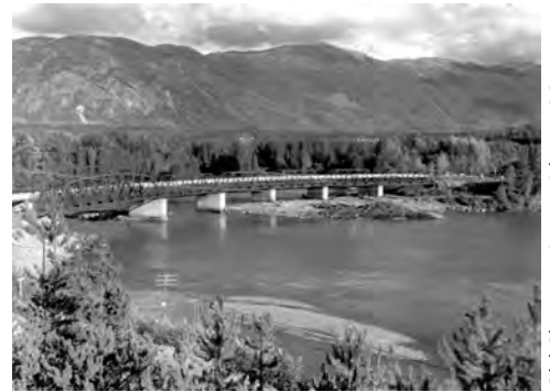
Old Skeena River Bridge, 1967. BCAR f-21880
