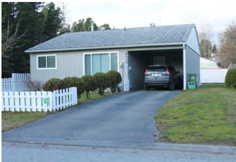
A SavMor house, part of Terrace's residential history.
