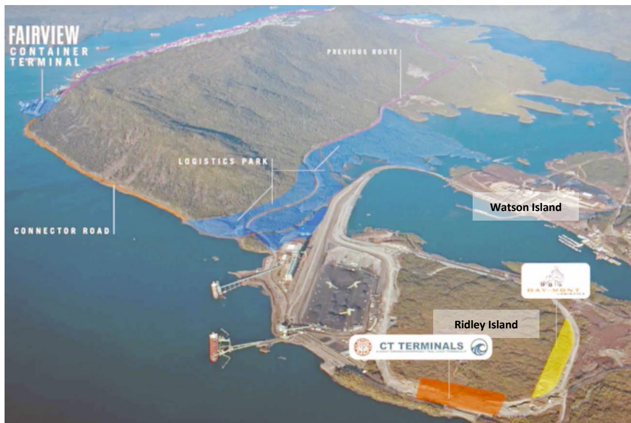
Figure 2-5: Fairview Container Terminal/Ridley Island Connector Road
