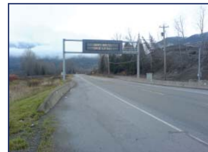
Section 3, as it currently exists, is occupied by Howe Creek for a section, and is generally characterized by dense brush, uncurbed highway shoulders and the raised rail bed to the south.
