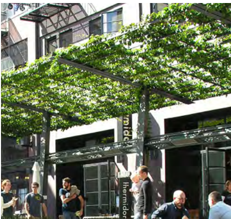
Landscape structures (e.g. arbors, archways, pergolas and trellises) that are integrated into the building may encroach onto the sidewalk
