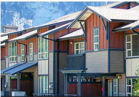
Building massing should be controlled in order to limit the impact of imposing forms
