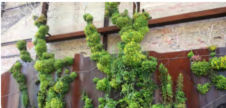
Where blank walls cannot be avoided as a function of internal program, opportunities for activation shall be explored
