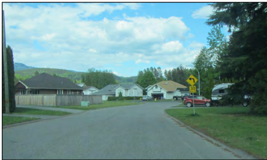
Figure 30: Local Road Example – Cooper Drive
