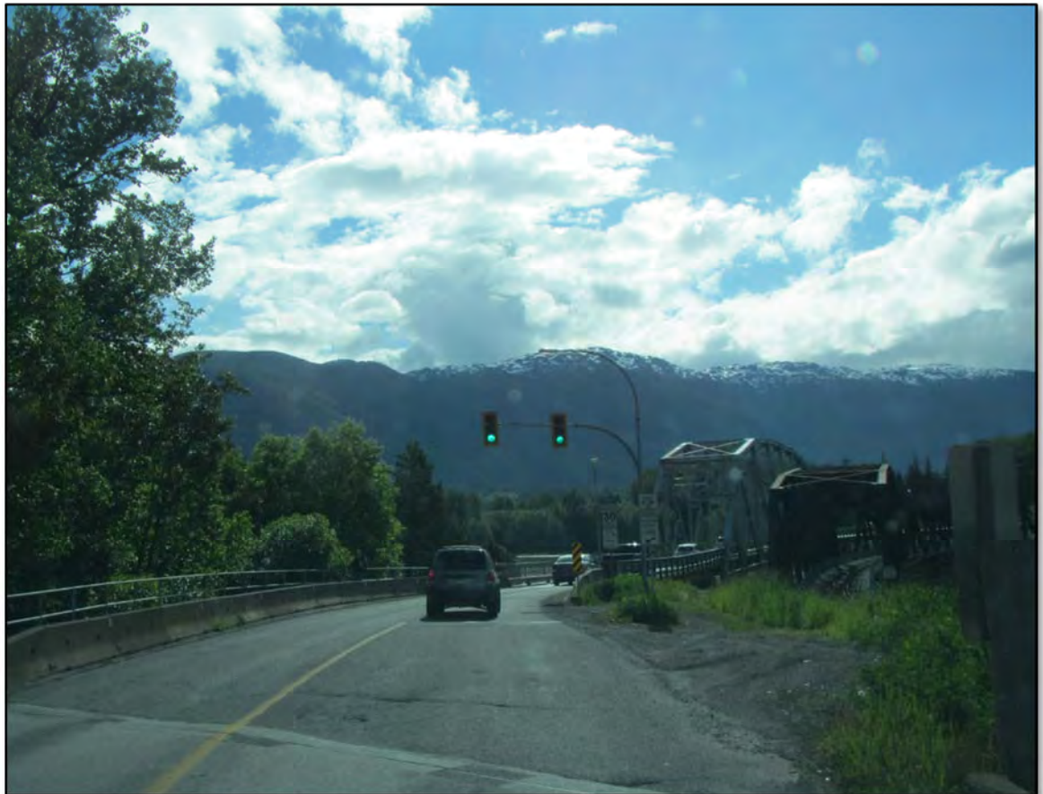
Figure 8: Old Skeena Bridge
