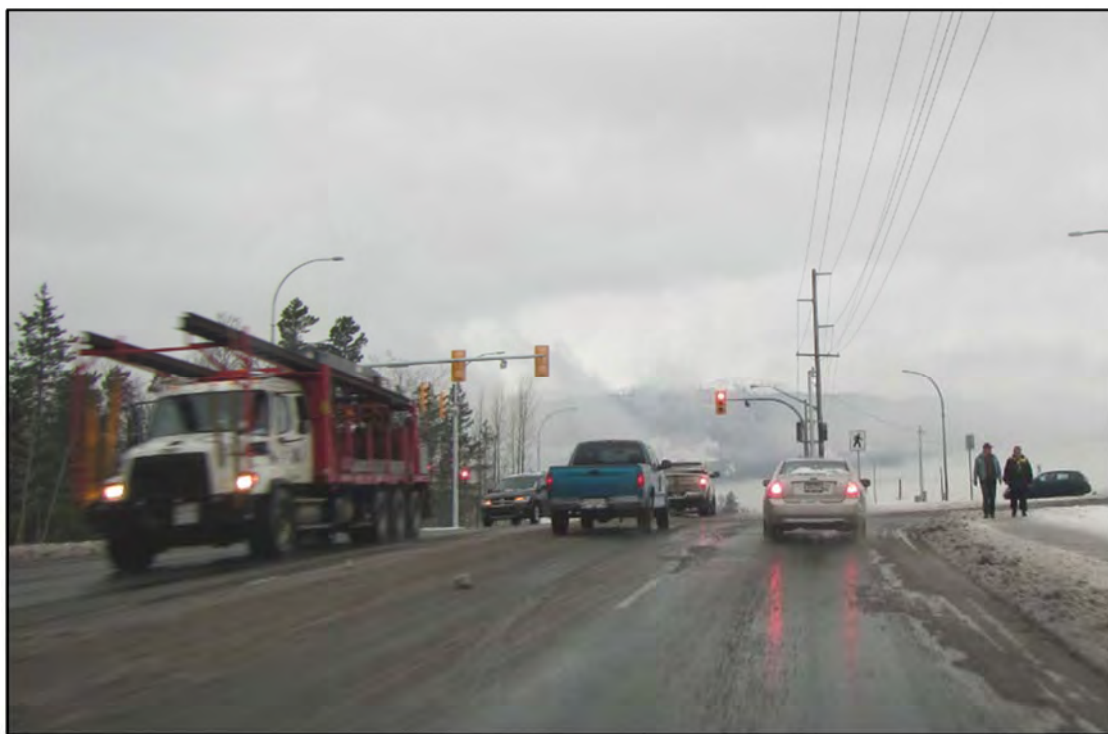
Figure 43: Highway 16 (Keith Avenue) at Sande Street
