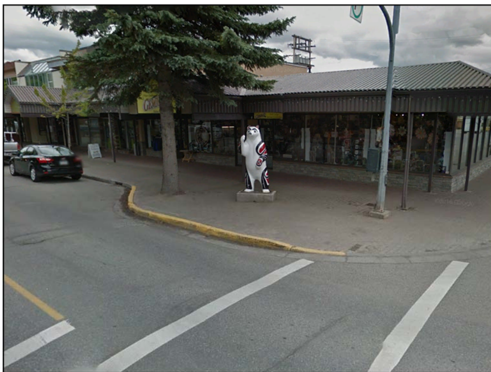
Figure 109: Sidewalk Bulb on Lakelse Avenue at Emerson Street
